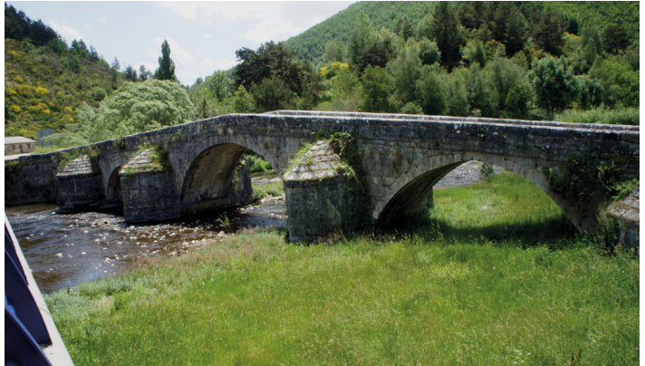
Photo: Boca de Huérgano Bridge (Lobo Quirce – Own work, CC BY-SA 4.0)
